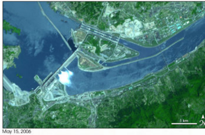
Figure 16. Aerial view of the Three Gorges Dam, China
