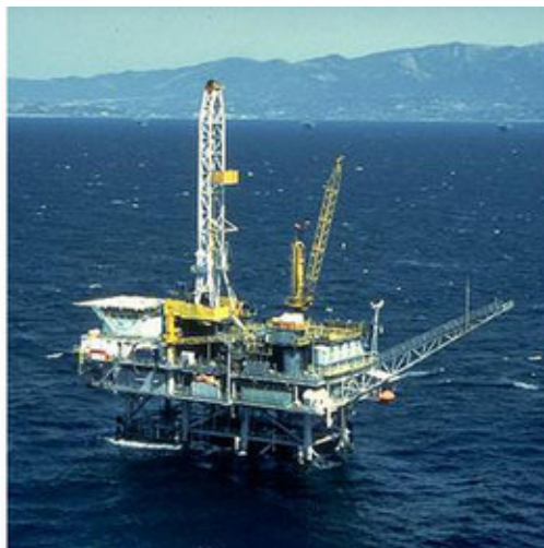
Figure 2. Offshore oil drilling platform, Gulf of Mexico
